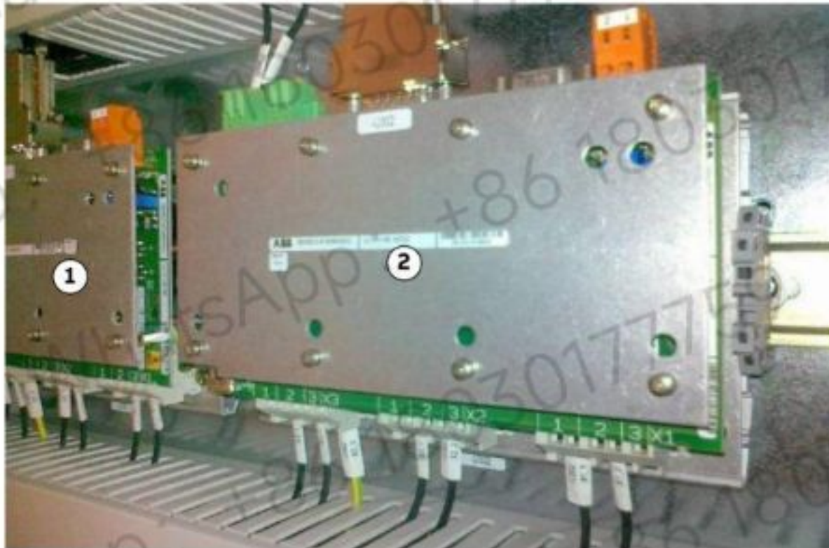
Figure 8-8 Voltage and current transducer boards UUD 148 AE01/2
