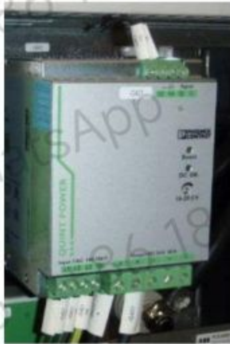
Figure 8-16 AC/DC converter Quint-PS/3AC/24DC/40
