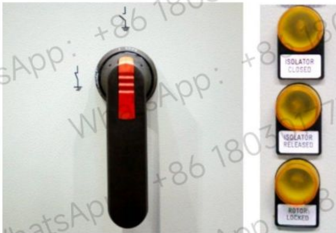
Figure 5-2 DC-link grounding isolator in position "not grounded"
