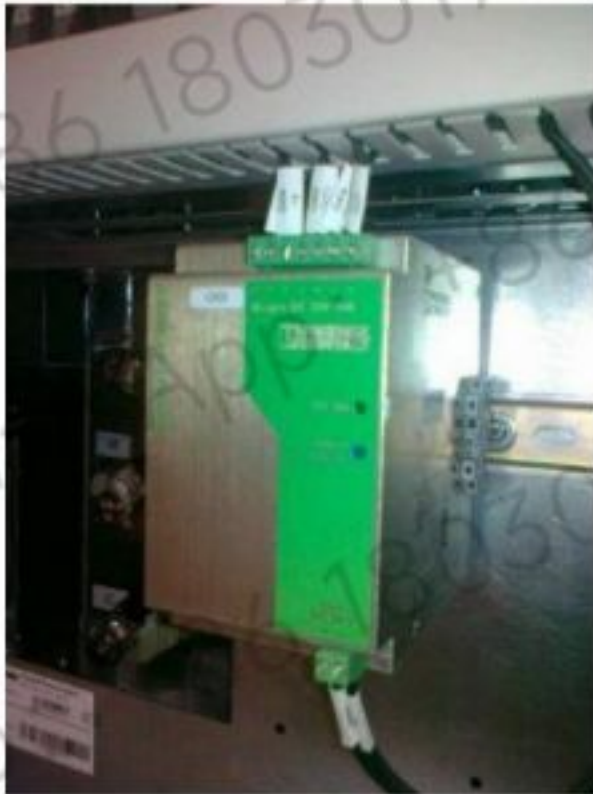
Figure 8–18 DC/DC converter Quint-PS-24DC/24DC/10
