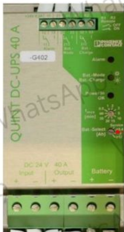
Figure 8-11 UPS -G402 selector switch "Bat.-Select"
