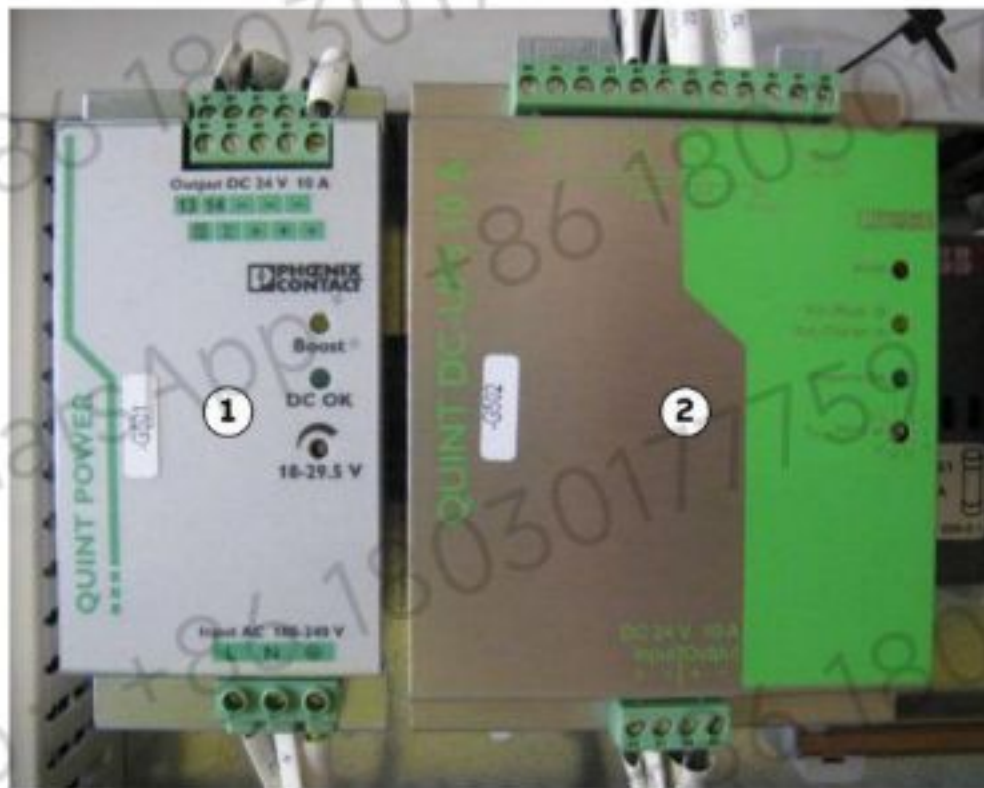
Figure 8-17 AC/DC converter Quint-PS/1P24/10
