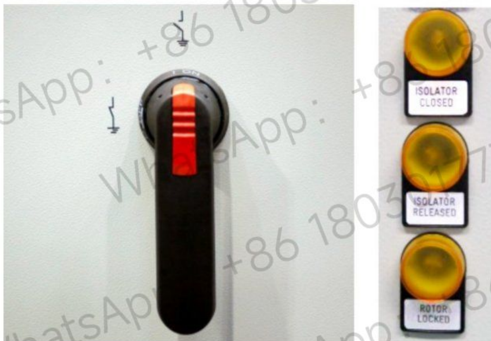
Figure 5-2 DC-link grounding isolator in position "not grounded"
