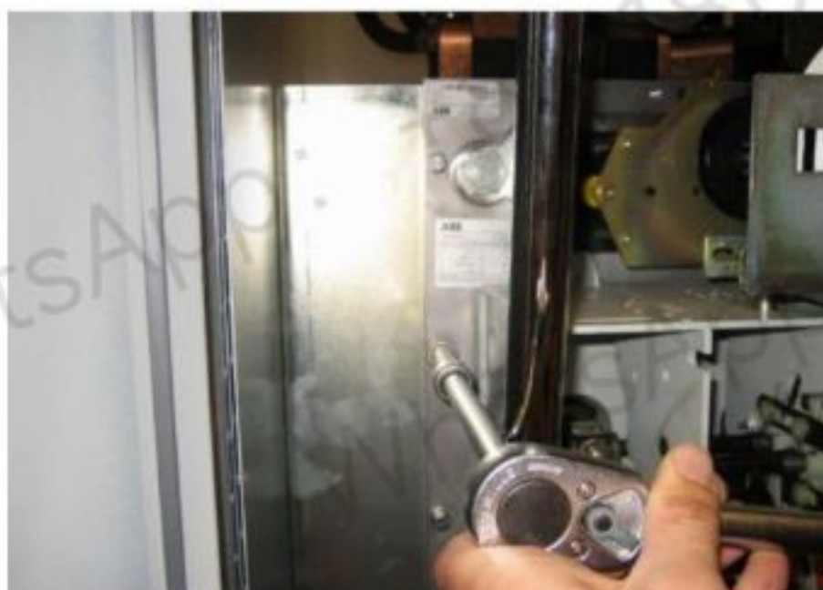
Figure 10-124 Unbolting the GEB
