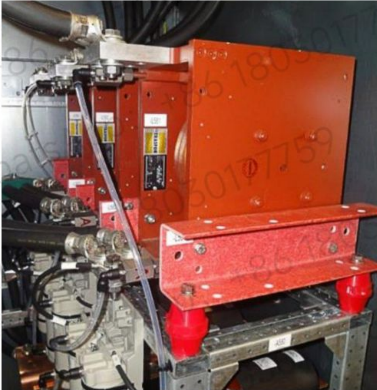
Figure 10–129 dv/dt filter reactor
