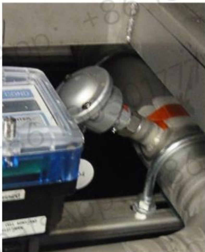
Figure 10–69 Temperature meter
