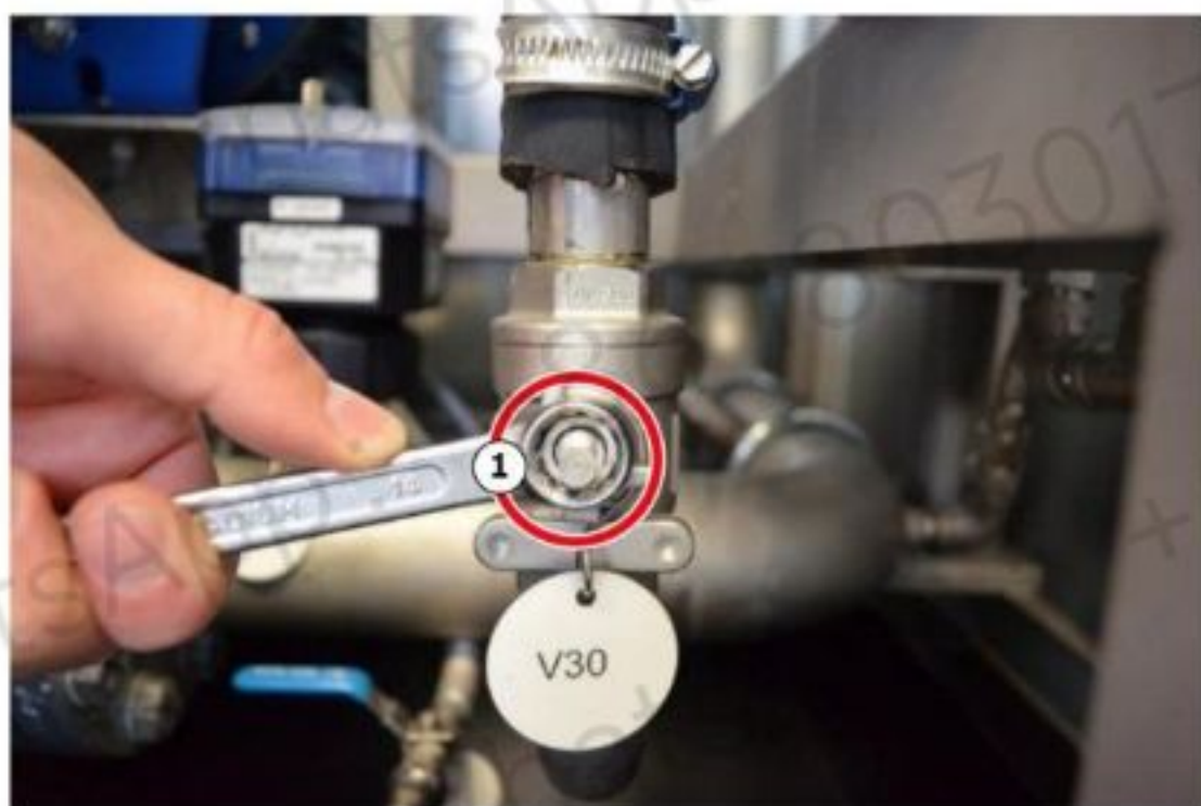
Figure 10-90 Gland from the Ball valve ¾"
