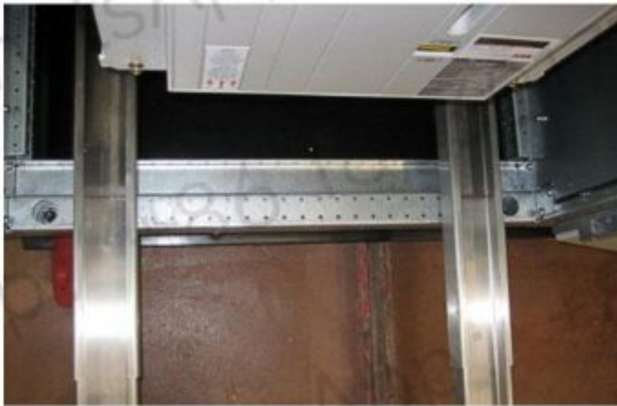
Figure 10-120 Trolley track beams (top view)
