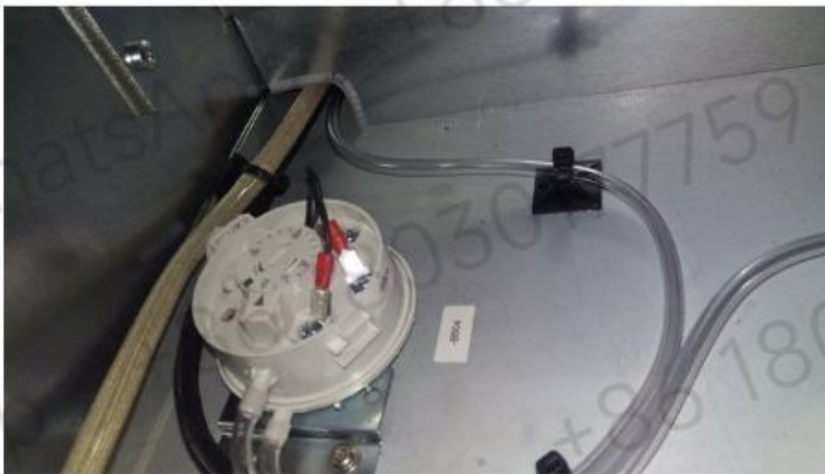
Figure 10-110 Differential pressure measurement device
