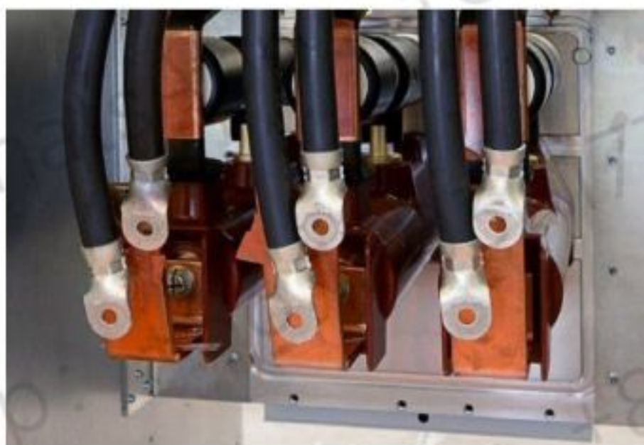
Figure 10-113 Breaker's lower power cable connections
