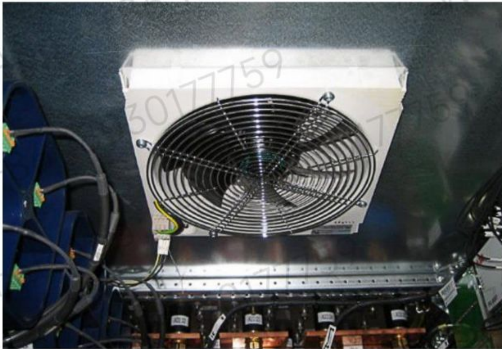
Figure 10–142 Roof fan
