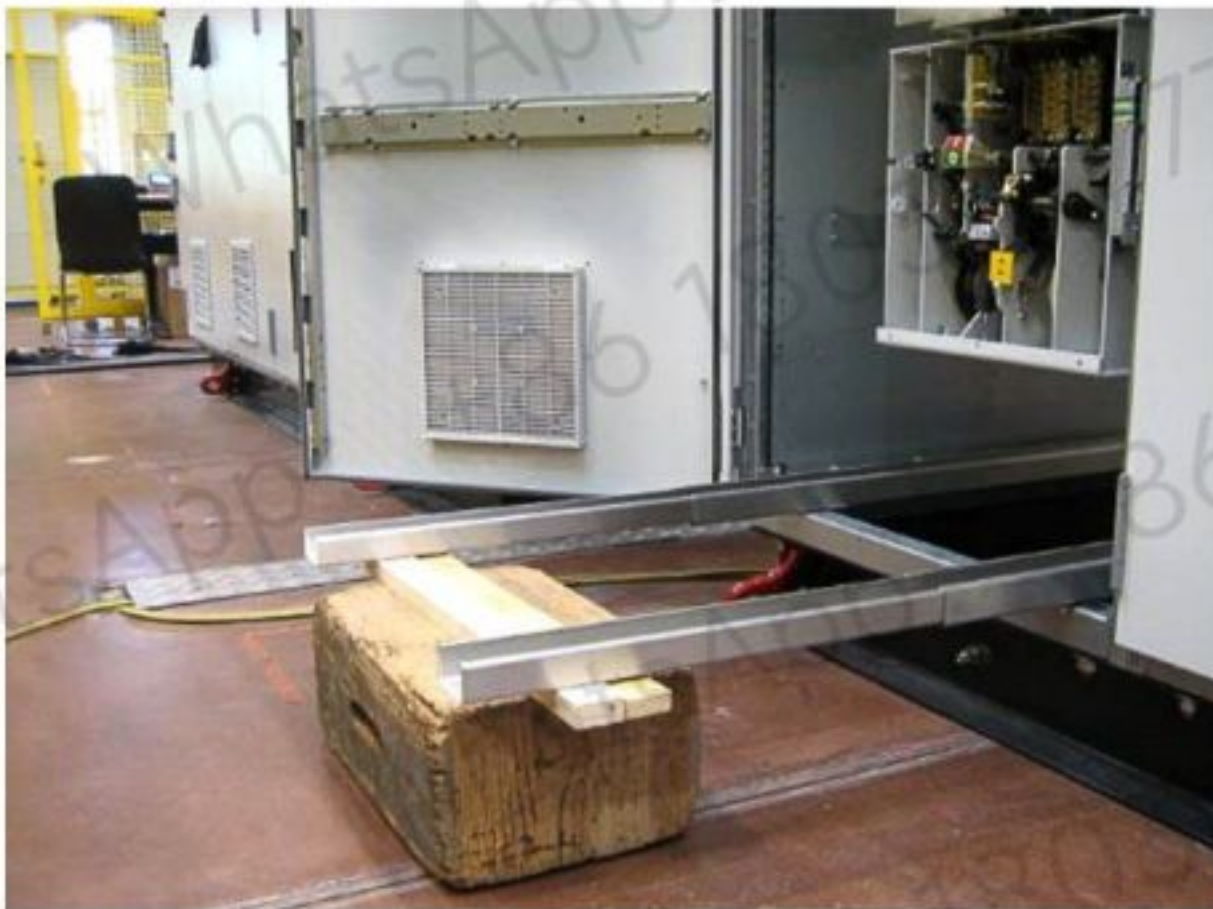
Figure 10-118 Trolley track beams
