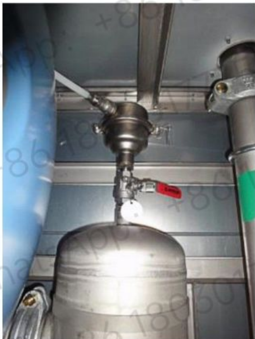
Figure 10–88 Automatic deaeration valve
