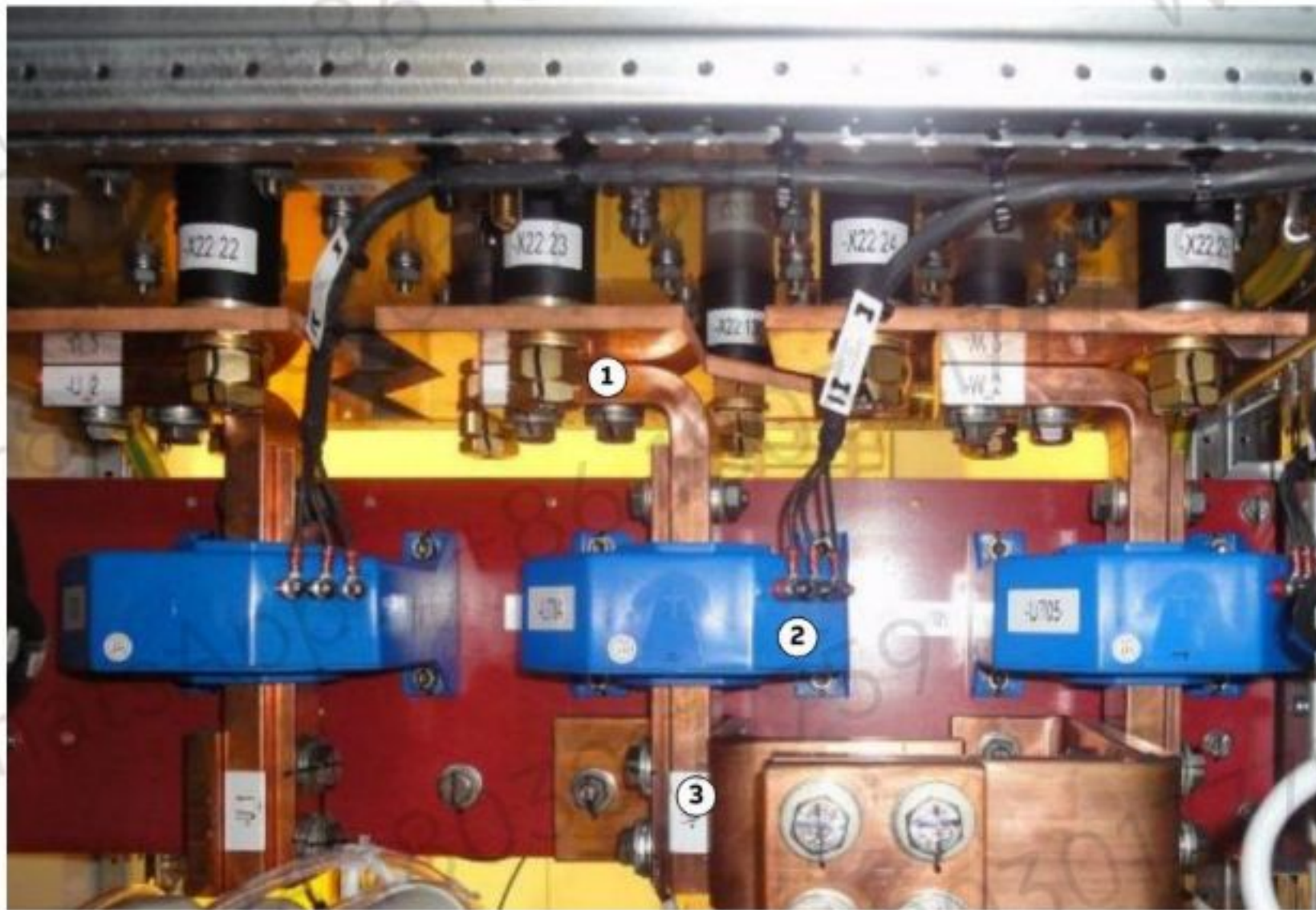
Figure 10-39 LEM current transducers
