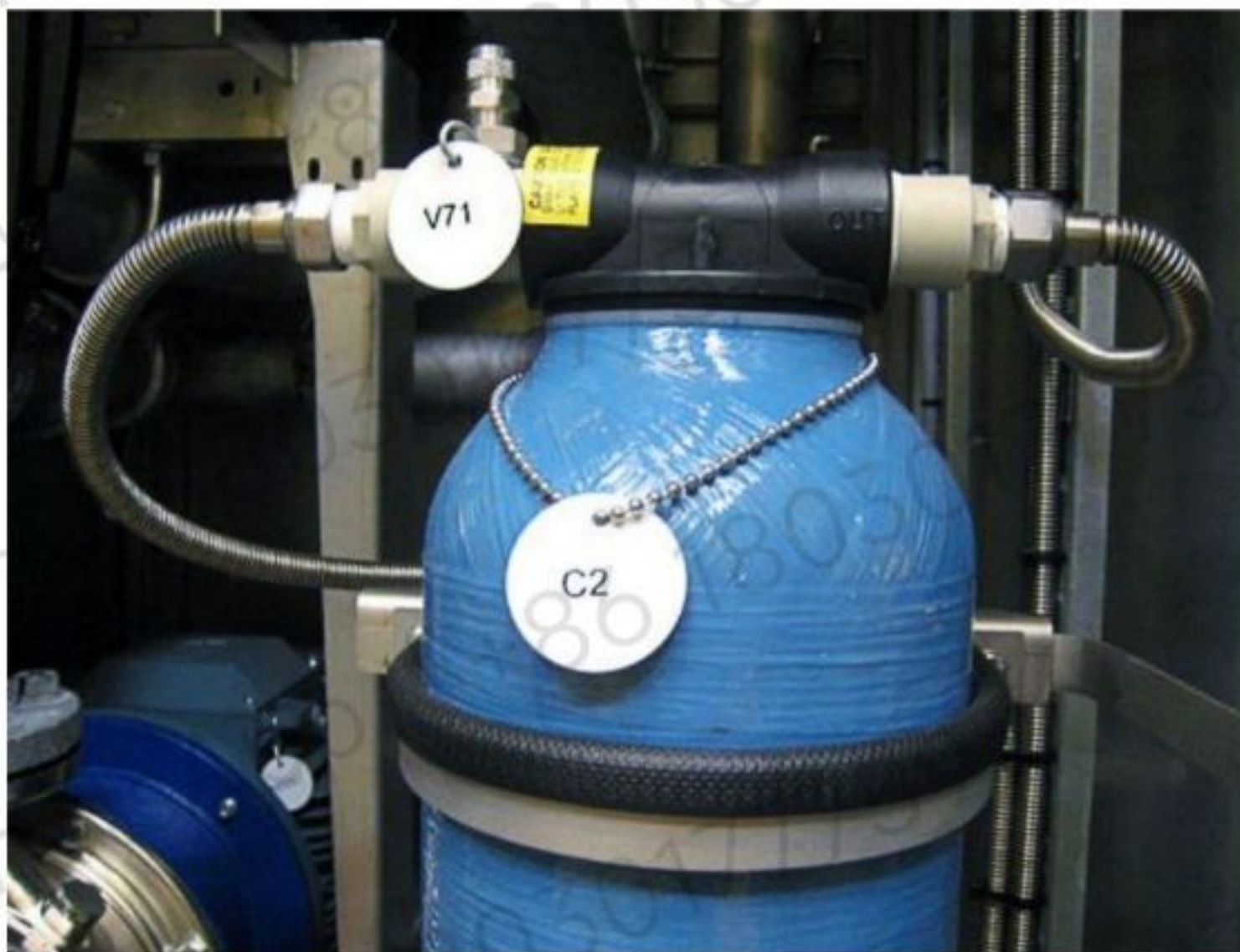
Figure 10-73 Ion exchange vessel
