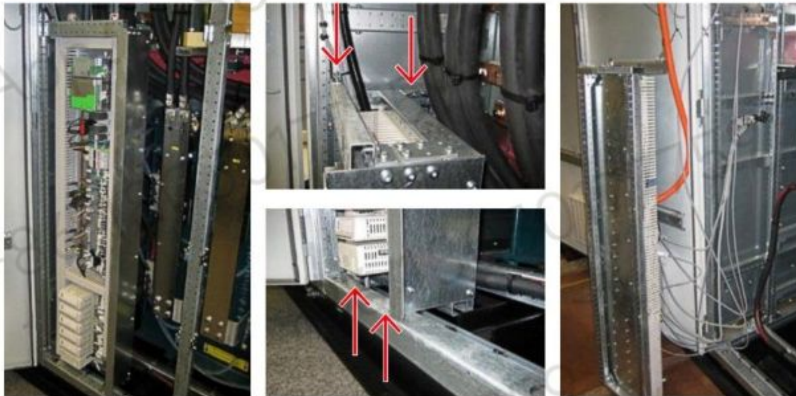
Figure 10–95 FCM removal (circles show bolt locations)
