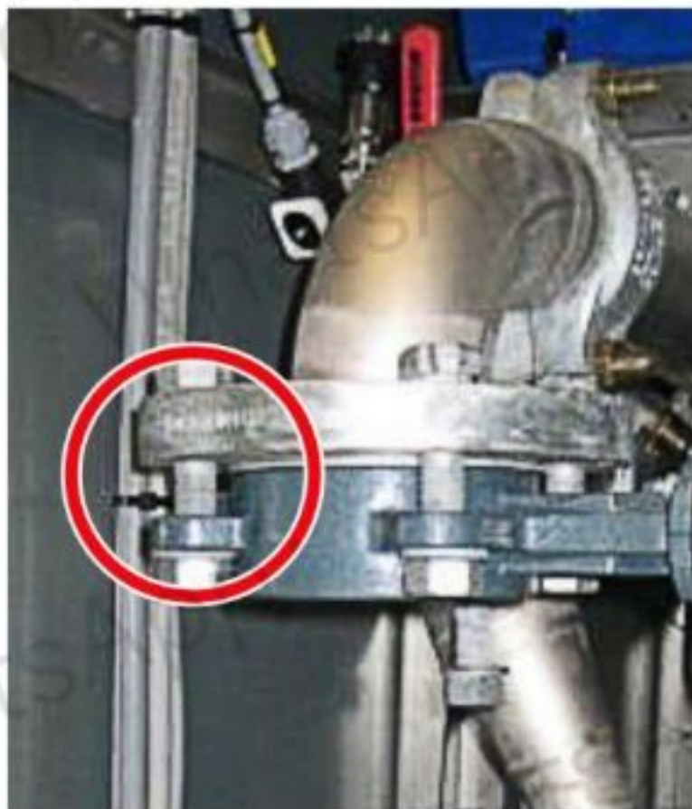
Figure 10-76 Pump flange
