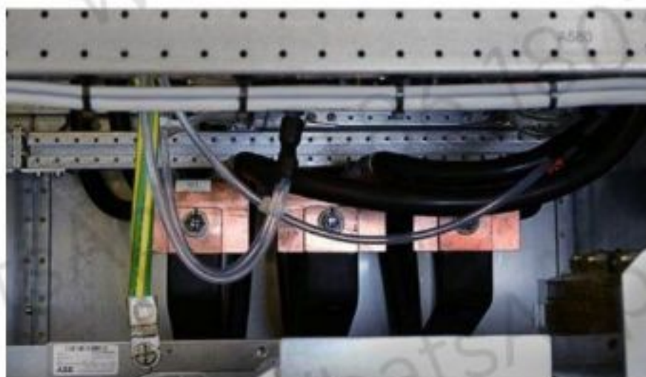
Figure 10-114 Breaker's upper power cable connection
