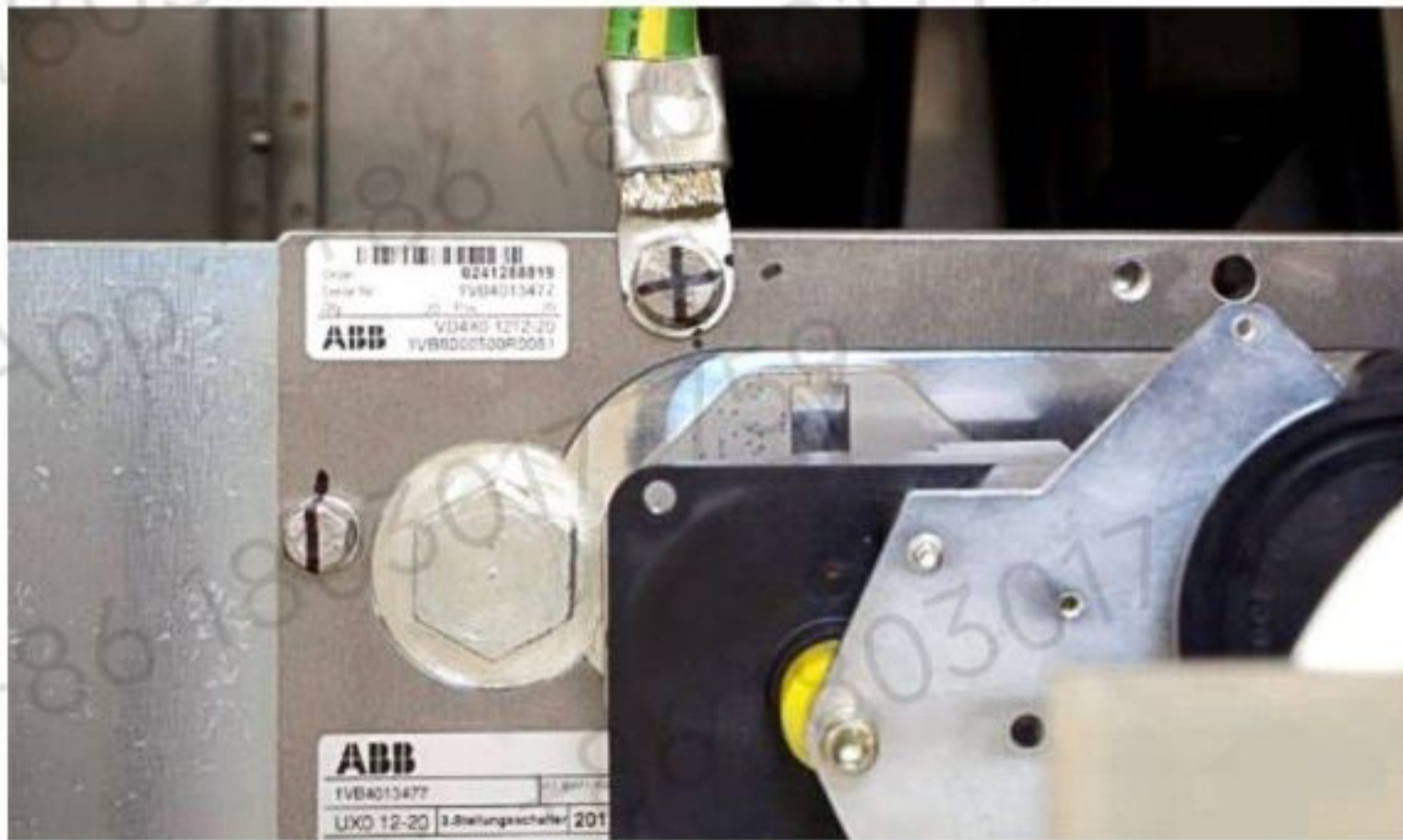
Figure 10-115 Breaker's protecting earth connection
