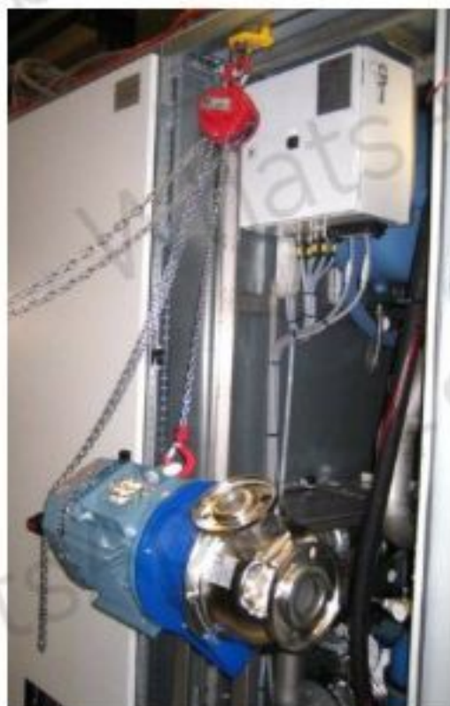
Figure 10–80 Use of chain-block to lift out pump
