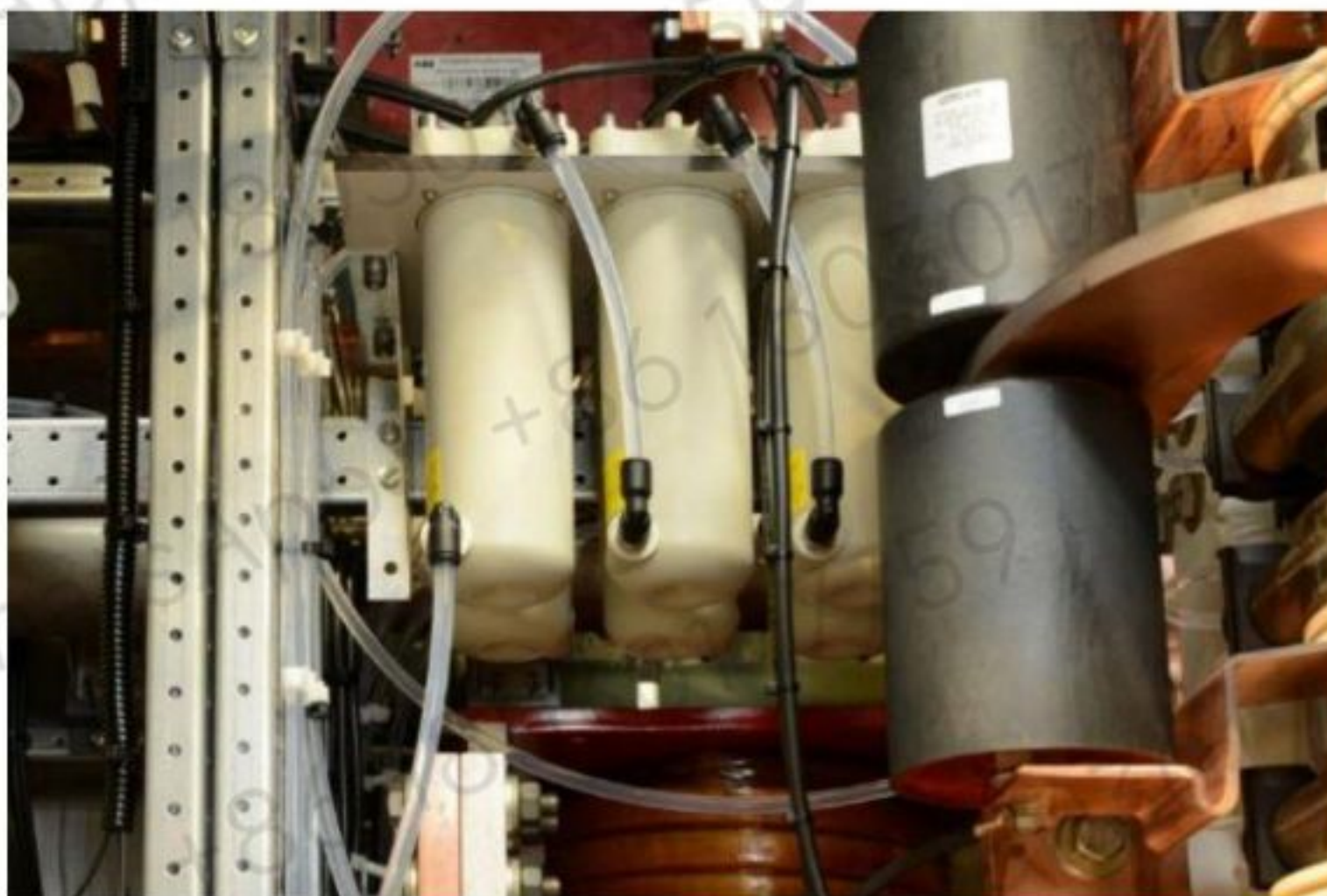
Figure 10–37 Clamp resistor
