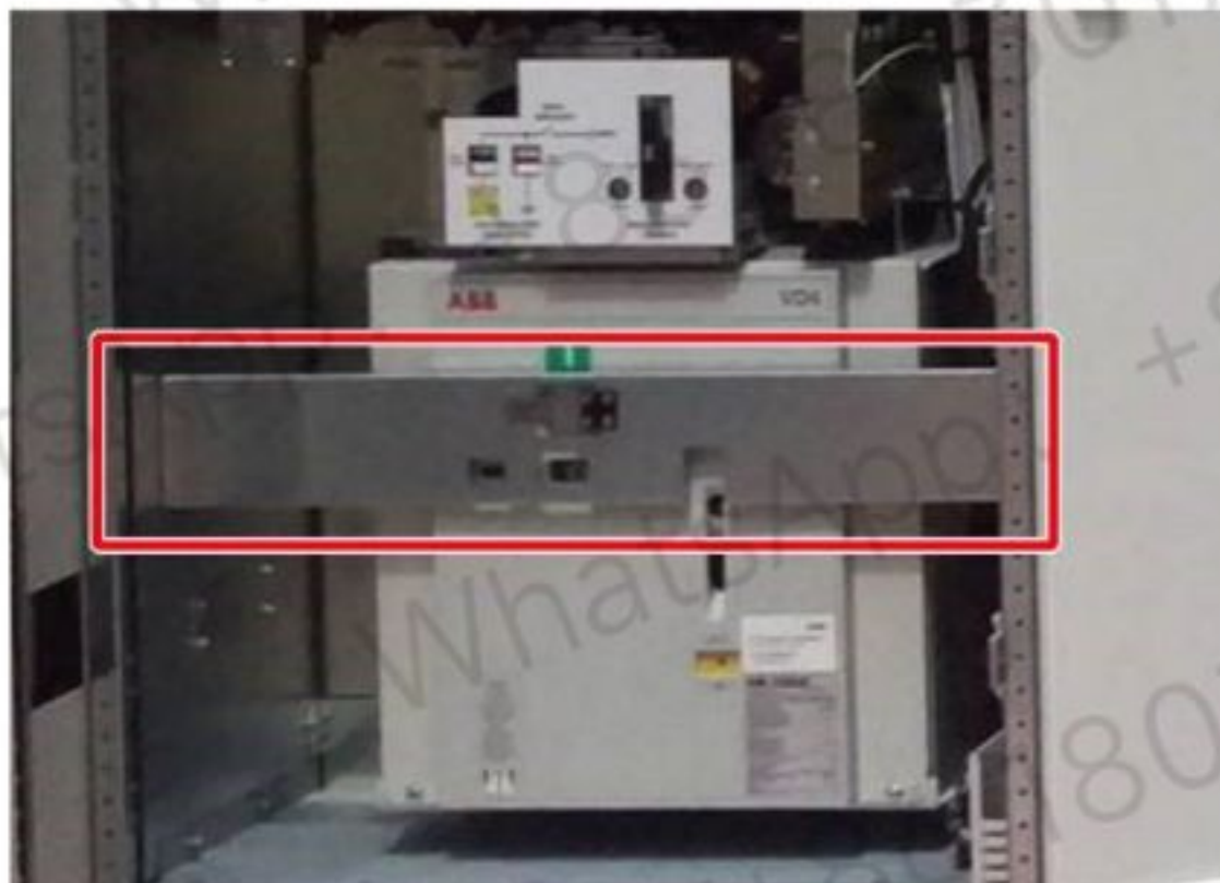
Figure 10-108 GBM push button locking device
