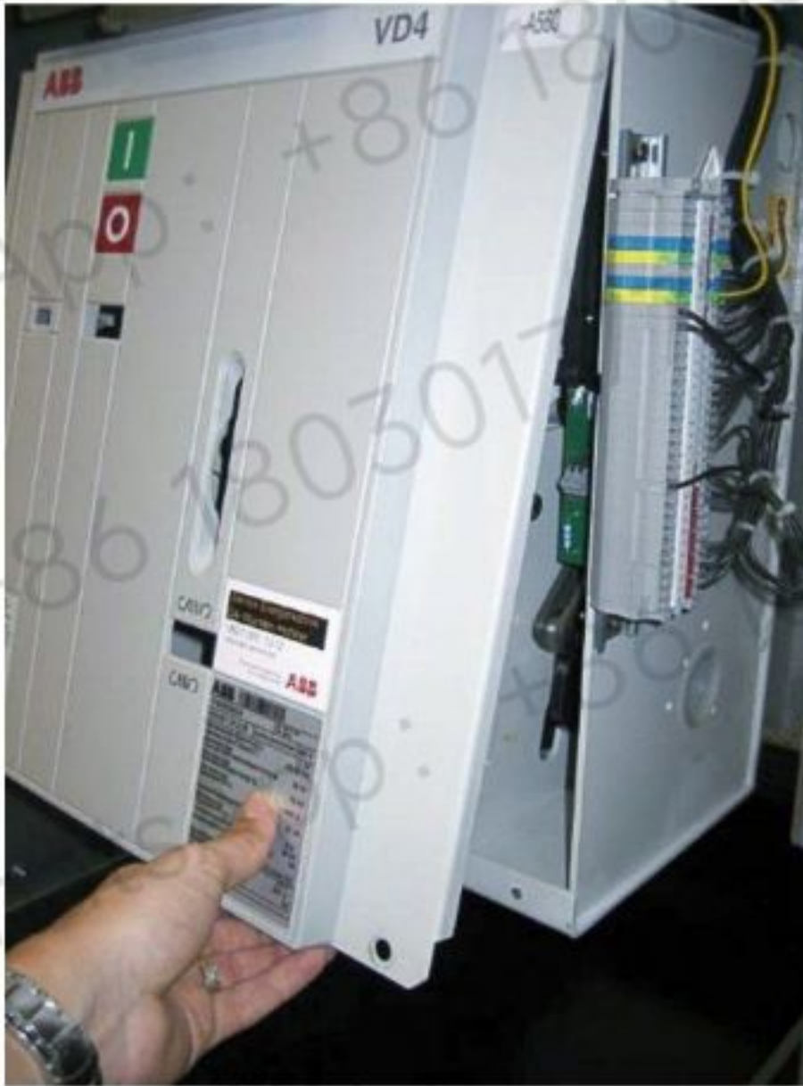
Figure 10-117 Breaker's protecting earth connection
