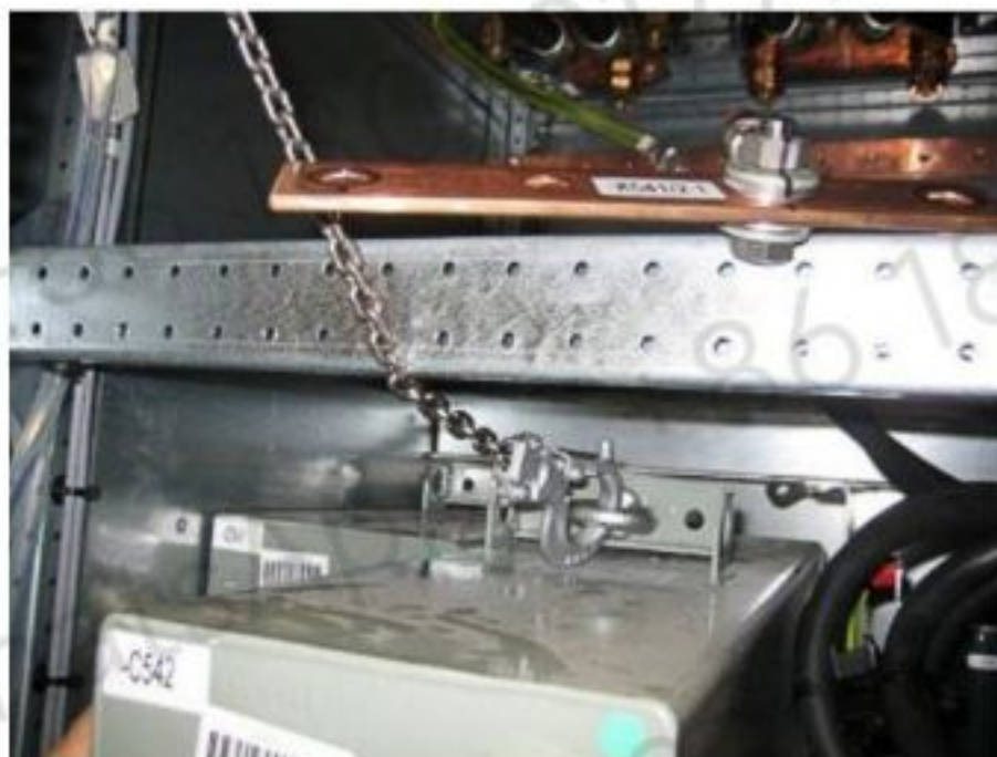
Figure 10–97 Lifting out capacitor
