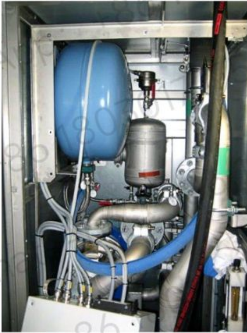
Figure 10-86 Expansion vessel
