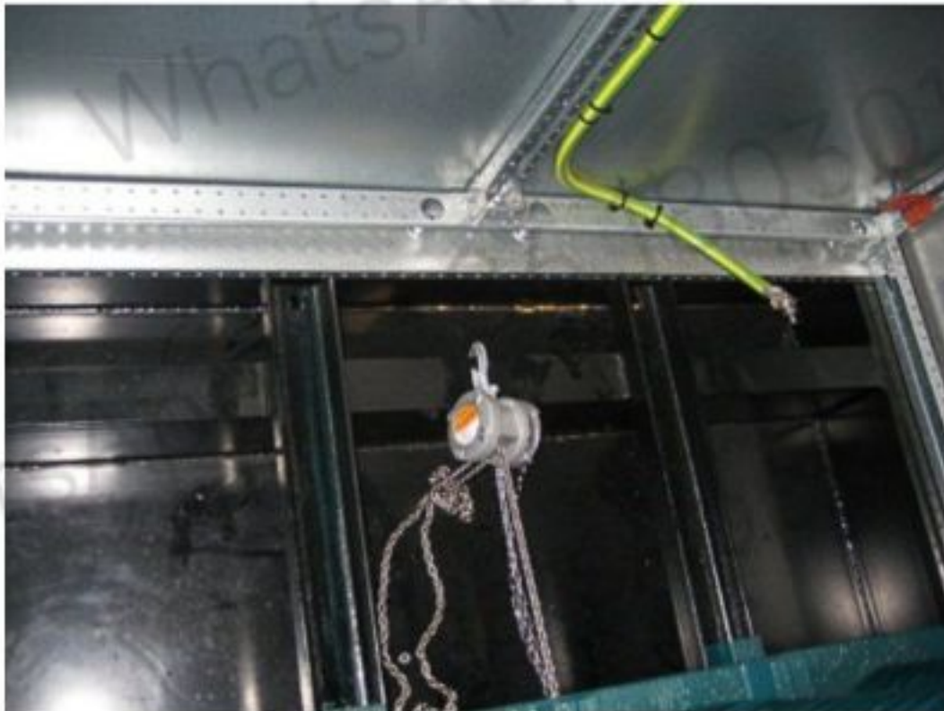
Figure 10-101 Ground connection
