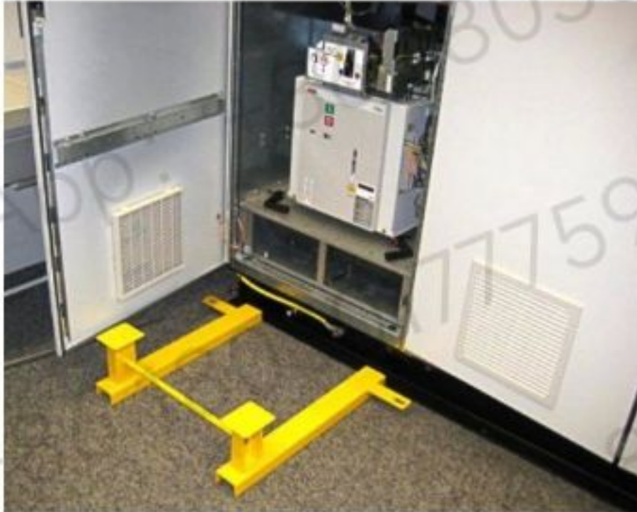
Figure 10-119 Support by reactor replacement kit
