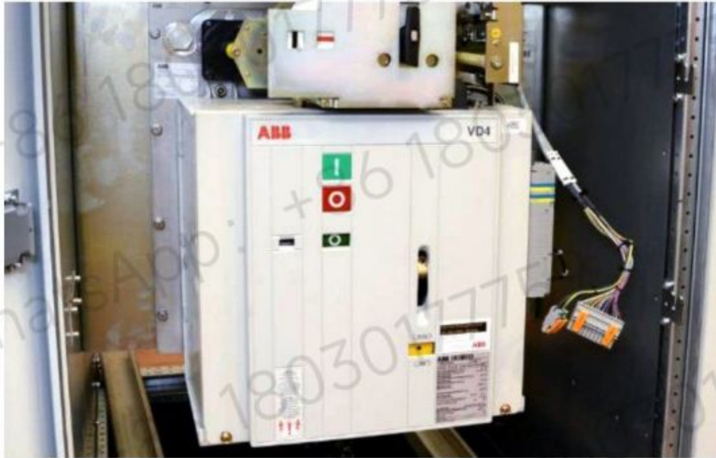
Figure 10-104 Generator breaker (GEB)
