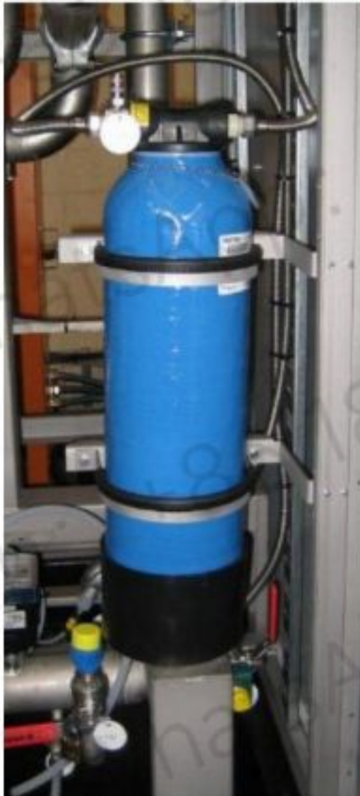
Figure 10–72 Ion exchange vessel (right side: old version)
