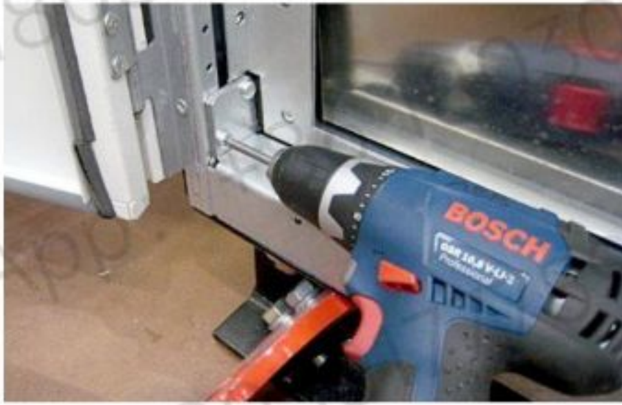
Figure 10-109 Lower front beam mounting screws
