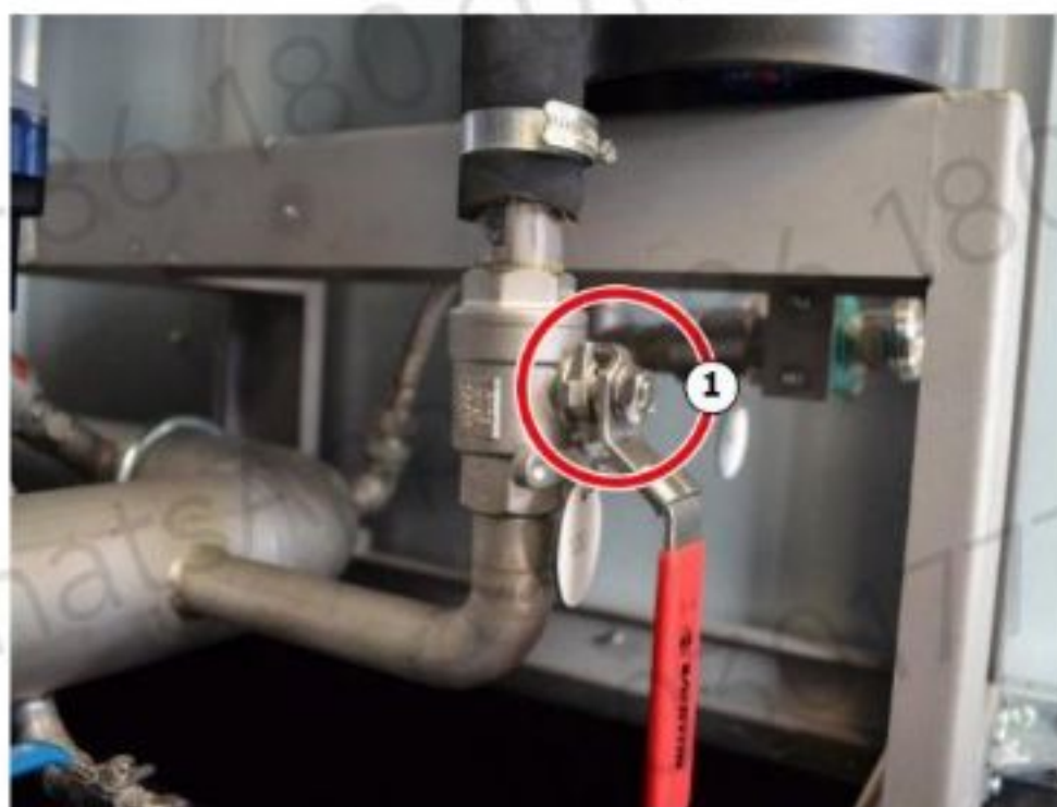
Figure 10-89 Ball valve ¾"
