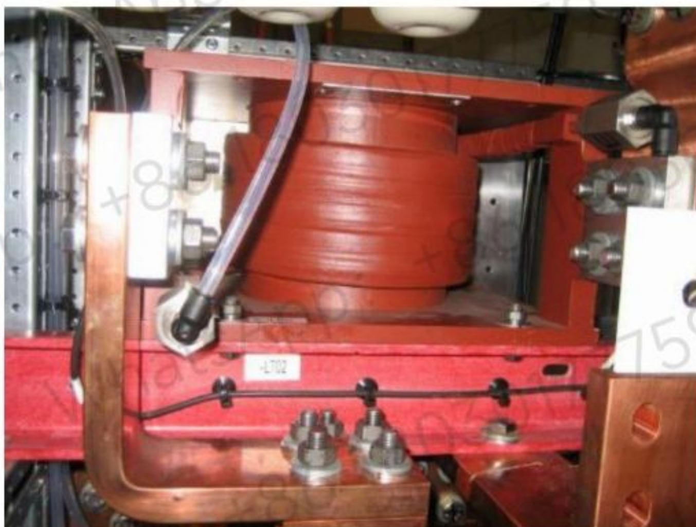
Figure 10–38 Clamp reactor
