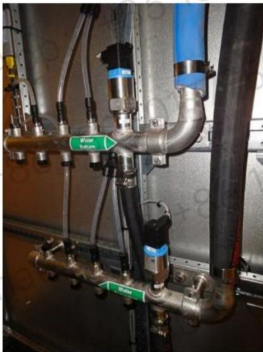
Figure 10–102 Pressure transmitter
