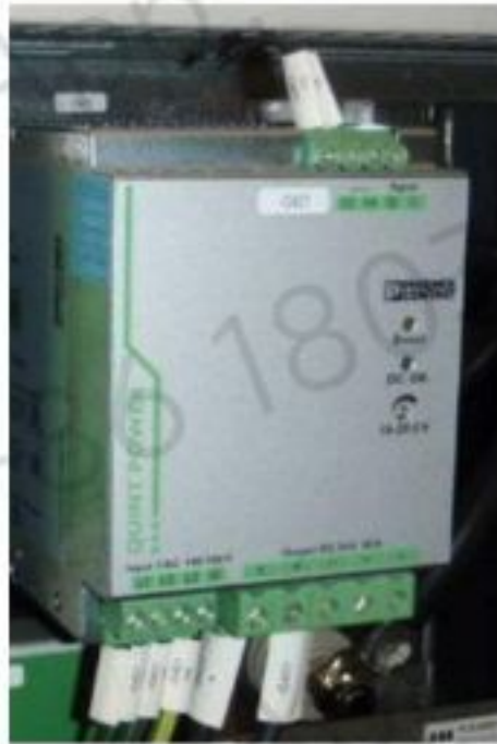
Figure 8-16 AC/DC converter Quint-PS/3AC/24DC/40
