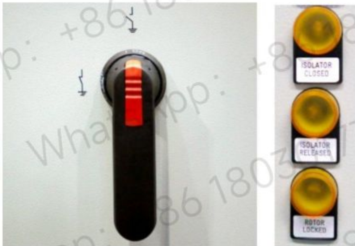
Figure 5-2 DC-link grounding isolator in position "not grounded"
