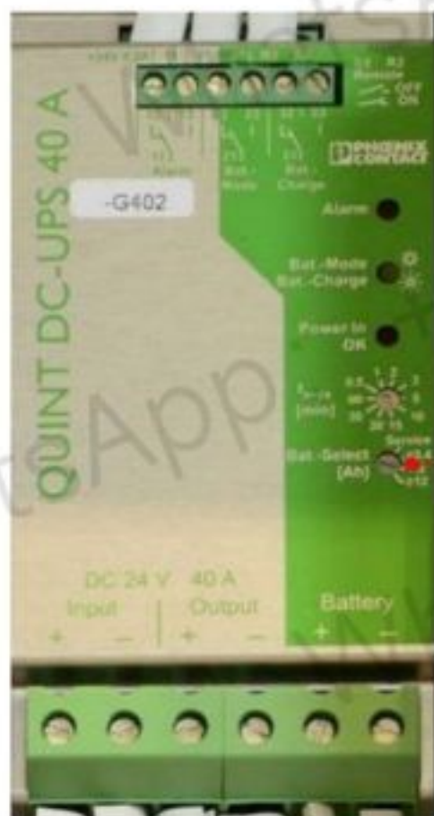
Figure 8-11 UPS -G402 selector switch "Bat.-Select"
