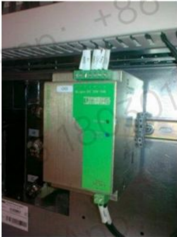
Figure 8–18 DC/DC converter Quint-PS-24DC/24DC/10
