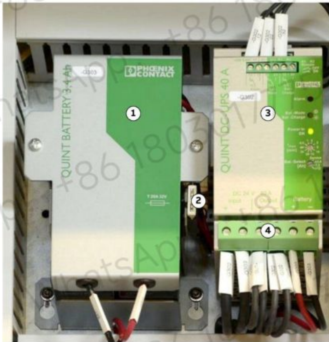
Figure 8-21 Battery -G303
