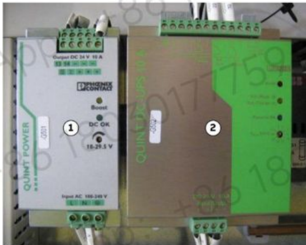
Figure 8-17 AC/DC converter Quint-PS/1P24/10
